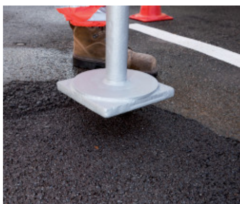
Compacting Mape-Asphalt Repair 0/8 by hand
