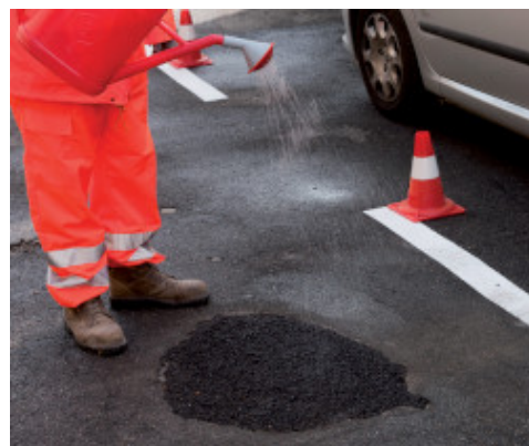
Wetting the surface of Mape-Asphalt Repair 0/8
