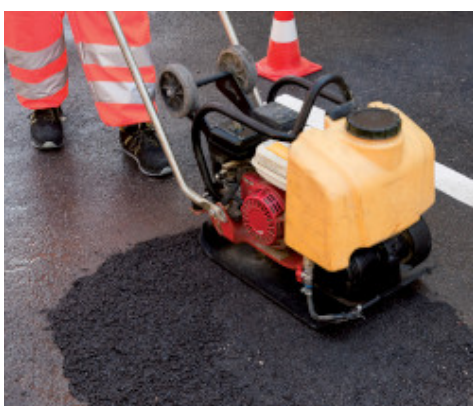
Compacting Mape-Asphalt Repair 0/8 with a vibro-compacting machine
