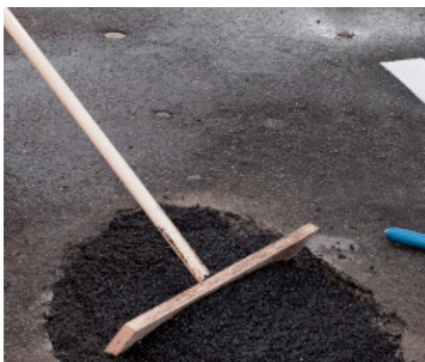
Applying and spreading Mape-Asphalt Repair 0/8
